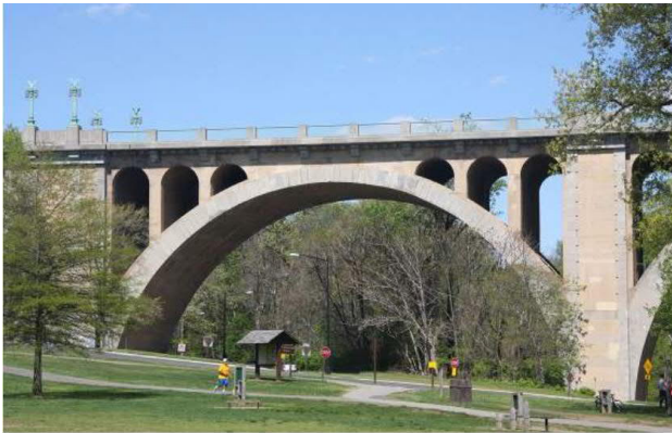
Under Bridge View - Rock Creek Park
