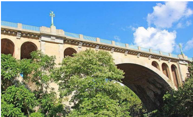
Under Bridge View – Rock Creek Park
