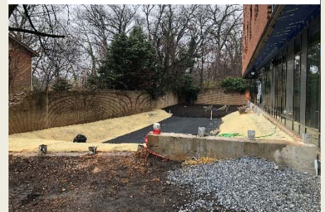
Bio-Retention Installation
