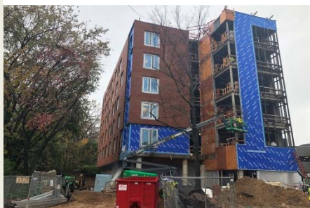
Brick Masonry Installation
