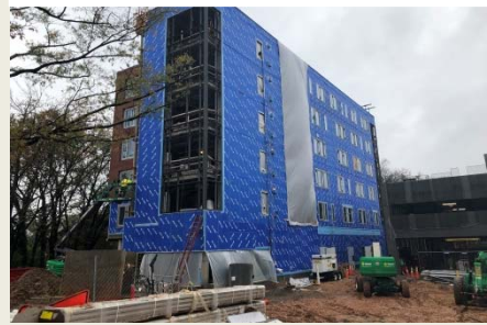
Curtain Wall framing installation
