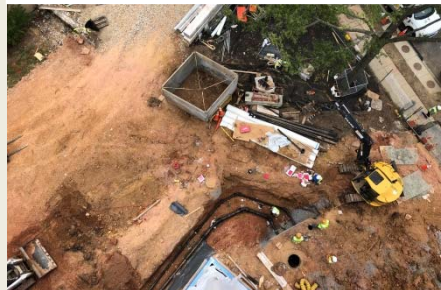
Site Utility installation
