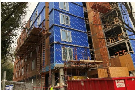
Brick Masonry Installation
