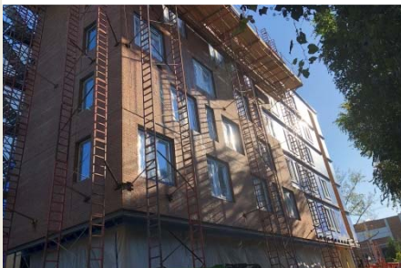
Brick Masonry Installation
