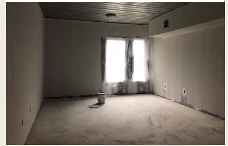
Unit prime in progress
