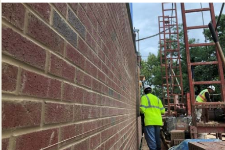
Brick Masonry Installation
