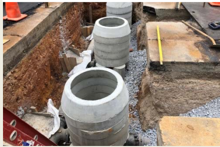
Site Utility installation
