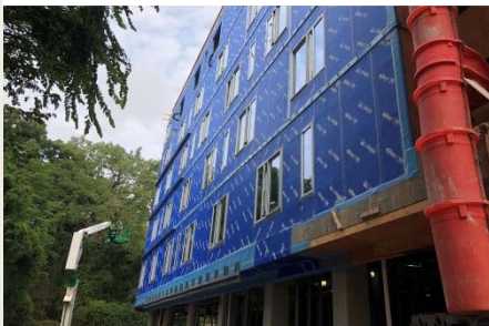
Window & Steel Angle Installation
