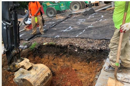
Excavation for Site Utilities
