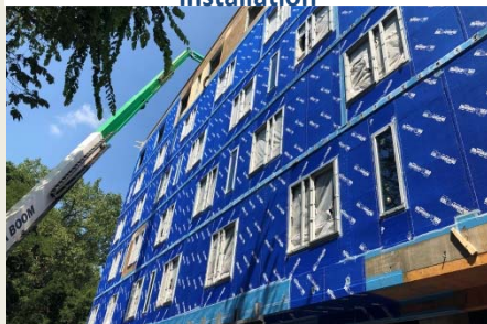
Exterior air Barrier & Window Installation
