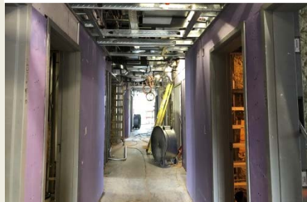
Drywall installation
