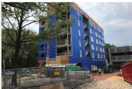
Exterior air Barrier
