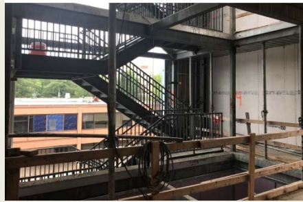
Metal Pan Stair installation
