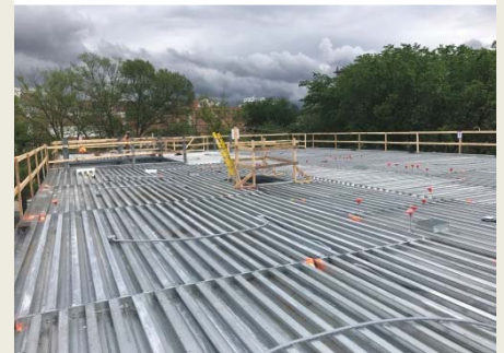
4 th fl. Elevated slab preparation
