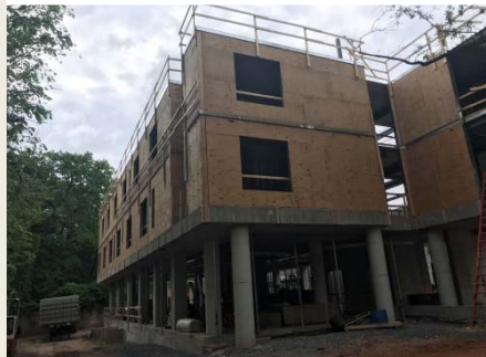
3 rd Fl. Structural Panels Installed
