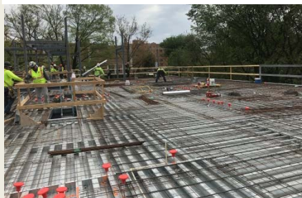
3 rd fl. Elevated Deck Prep
