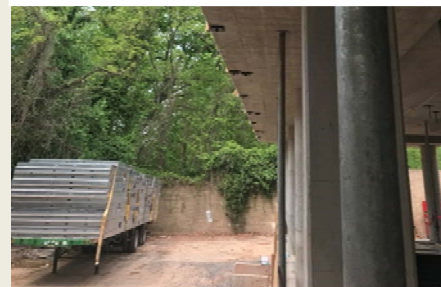
3 rd Fl. Structural Panel Delivered
