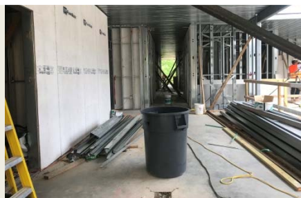
Structural Panels @ Podium Slab
