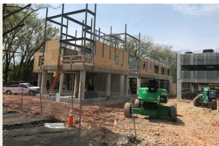
Structural Panels @ Podium Slab
