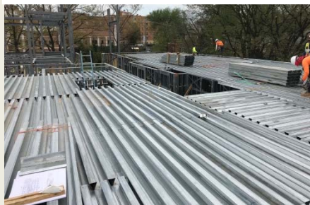
Metal Deck Installation
