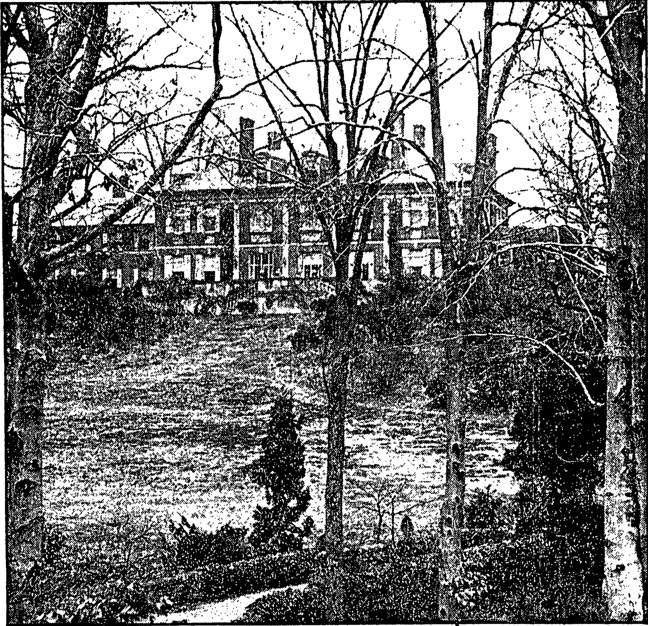
The 24-room mansion of the Tregaron estate, seen from the rear.
